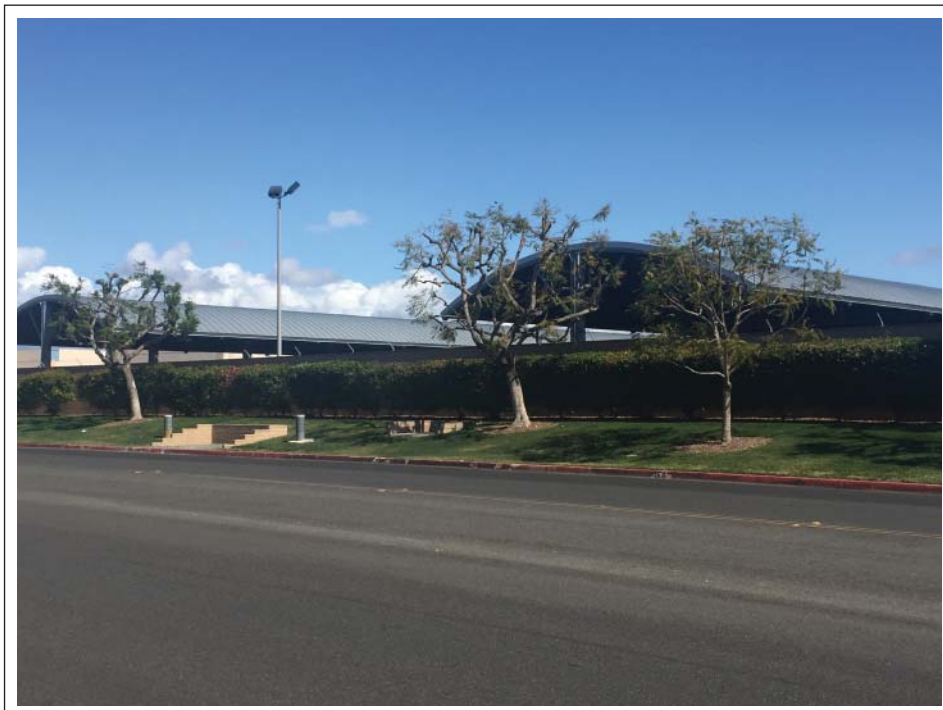
Photograph B: Airway Avenue, north of Baker Street, looking northeast.
